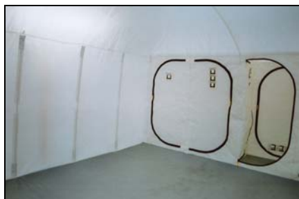
Powerply CW & BW agent resistant liner. Note the airlock design.
